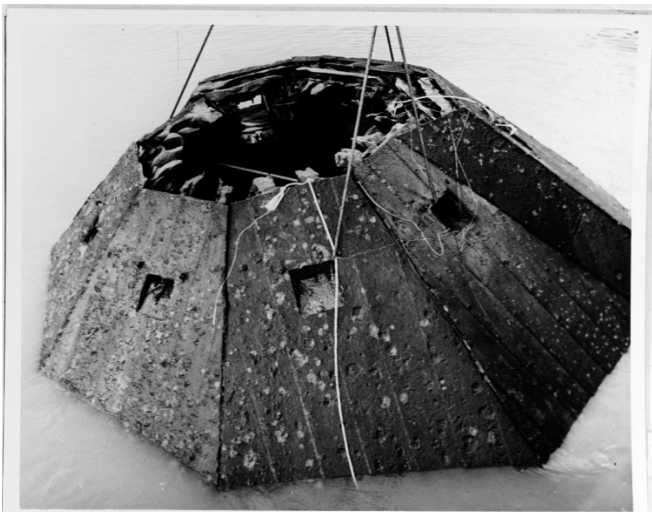
The pilothouse being removed from the river. Of particular note is the extra armor added to the front of the housing which faces the upper right of the photo. After action at Forts Henry and Donaldson by other
