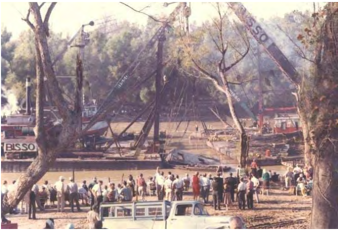
Raising the ironclad didn't go as planned. As the barges lifted the hull, the cables began to cut into the hull. Rather than letting her break apart, Cairo was intentionally cut into pieces and placed on the barges. Here we see the forward part of the casemate breaking the surface. Also notice that the Yazoo isn't a particularly wide river (est. 100 yards) at the point of the sinking. This made maneuvering the salvage craft difficult.
