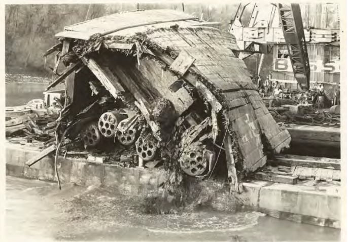
Central portion of the hull showing the end of the firetube boilers. This section rotated 90 degrees during the lift and had to be placed on the barge on its side.
