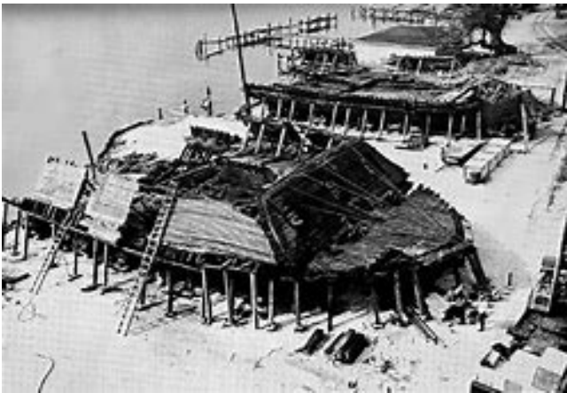
Cairo after being sectioned and raised. This is while in storage at the Ingalls Shipyard in Pascagoula, MS
