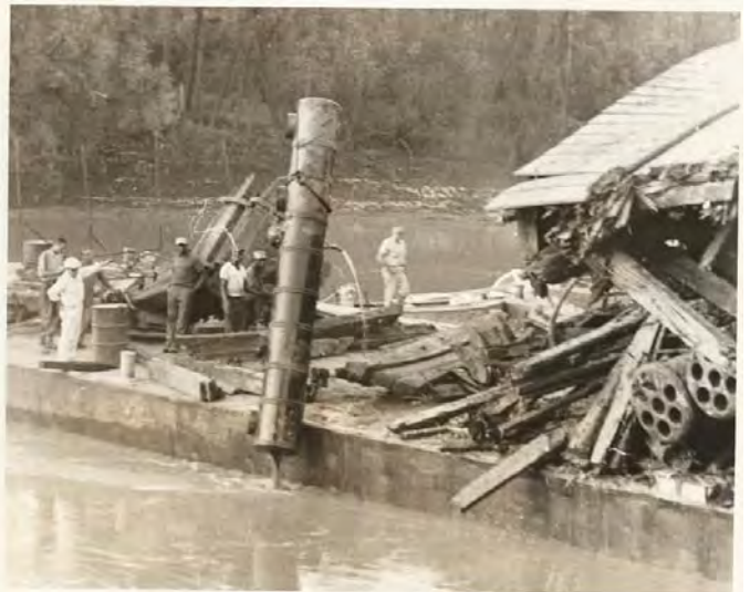
This appears to be the condensing tank that sat atop the boilers and allowed the steam to cool before it was re-circulated into the boilers. This is almost certainly taken at the same time as the preceding picture.
