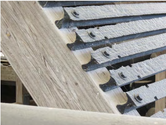
The rails were mounted with the top of the rail inward and the wider base facing outward. I wonder about the spacing as there are nearly two inches between the rails in this photo. Perhaps being mounted at an angle gave the effect of closer spacing and would let them get away with fewer rails used in each location.
