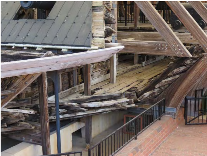
The spot at the corner of the casemate where the torpedo exploded. Note the mix of original wood supported by a modern, laminated frame. They have made an effort to be clear what is new and what isn't.
