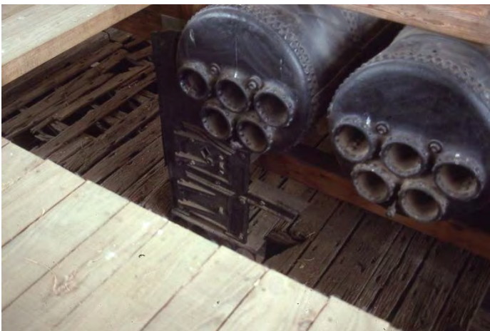
One of the fire doors for stoking the firebox with coal. Coal was preferred as it was more energy efficient versus wood but it had to be shipped in versus simply sending men ashore to cut down trees. This is the only one displayed but there would have been more in order to have a balanced burn. The coal bunkers would be nearby. The coal bunkers were also located so to act as additional protection.
