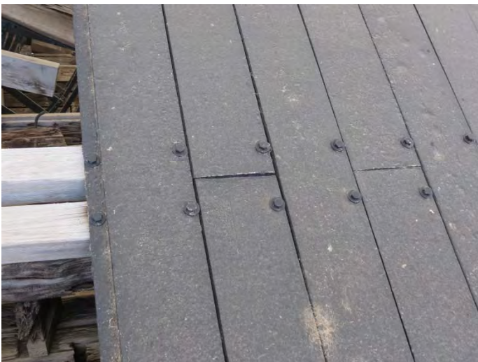
One thing that surprised the salvagers was that the plate wasn't butt-fitted but tongue and groove. I was then also surprised that the bolt
