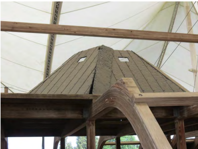
A clear illustration of how the extra 'spaced' armor was applied to the face of the pilothouse.
